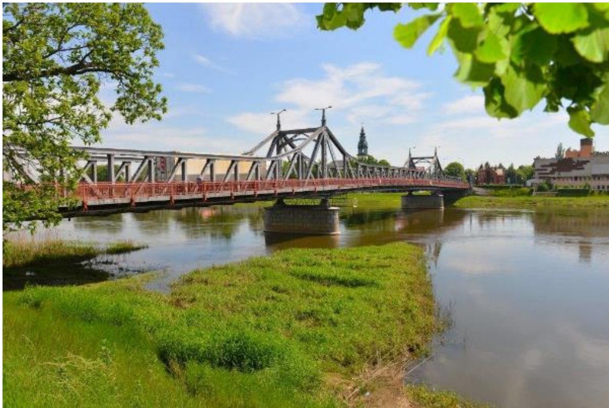
Phot. 1 The existing bridge in Krosno Odrzańskie.
