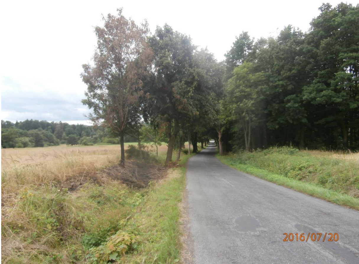
Figure 8 – Section of district road No. 3233D located in the area of the right bank abutment of the dam, western view.
